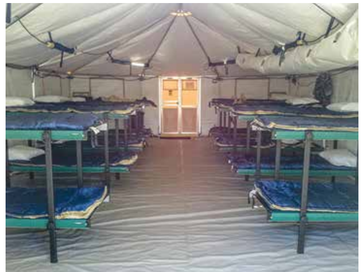
Shelter billering featuring Western Shelter bunk beds, air distribution plenum, lighting and wiring harness.
